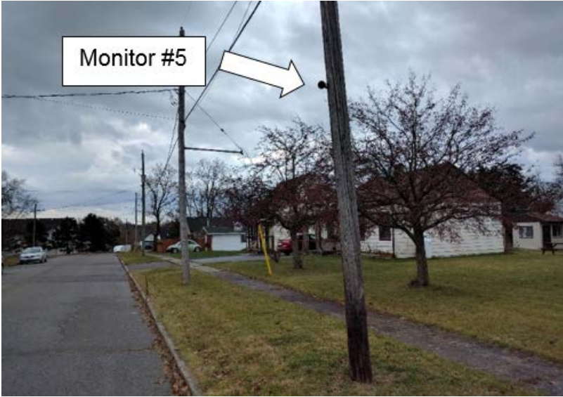
Figure 5. Noise Monitor Set-up at 64 Delany Ave. (POR #2)
